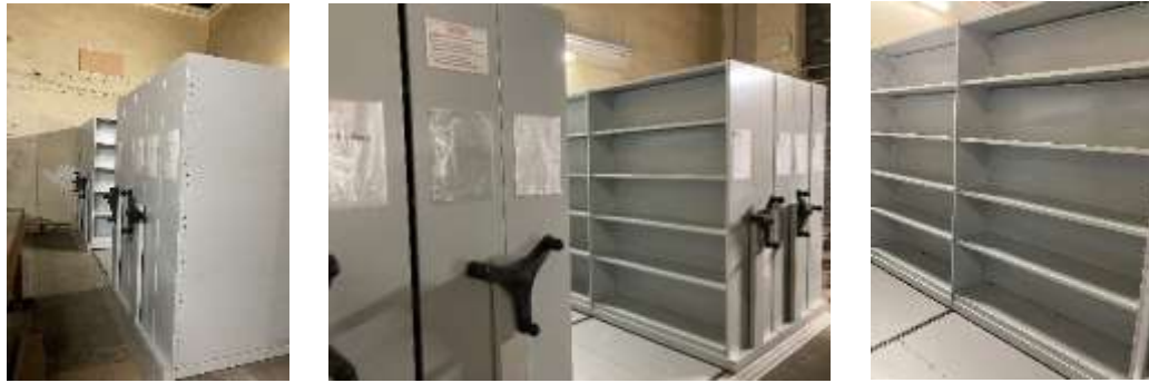
Images of the reinstated archive storage units
